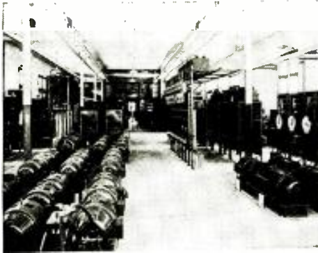
THE PALO ALTO STATION One of the powerful Mackay Radio inter-city radio telegraph stations—near San Francisco.
